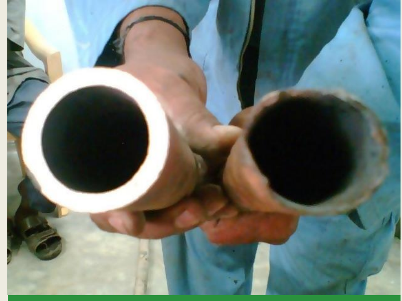
Corrosion On Super Heater Tube (Gas Side)
